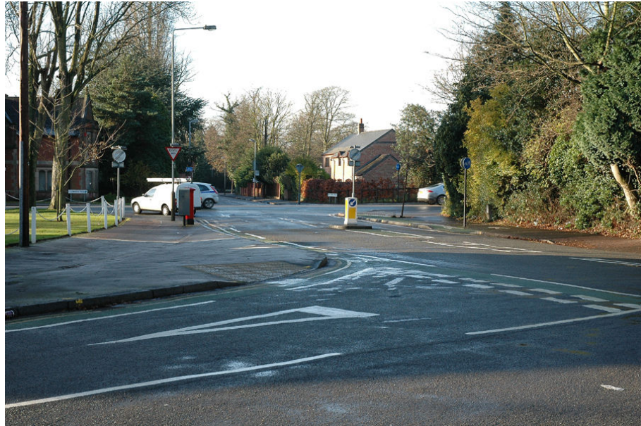
Fig 10. Manor Road/Guildford Road/London Road junction (looking west)
